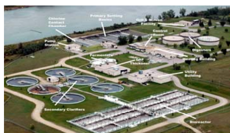
Figure 6.4.1 A Typical Biological Sewage Treatment Plant
